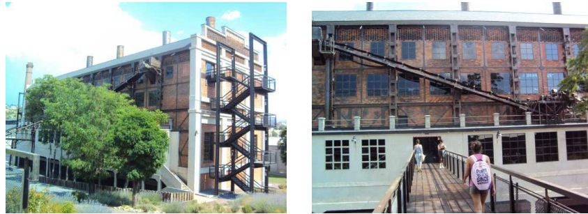
Figures 12,13. The Museum of Energy (Fábrica de la Luz), Ponferrada, Spain, in a former central thermal plant, exterior views (Source: photos by the author, 2013)
