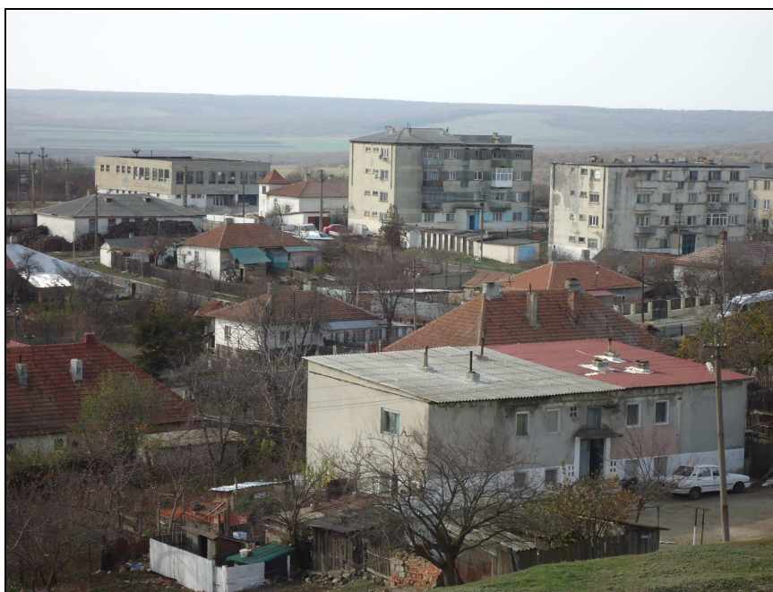
Fig. 6. Altân Tepe – abandoned housing service, Minvest S.A. (November 2015)
