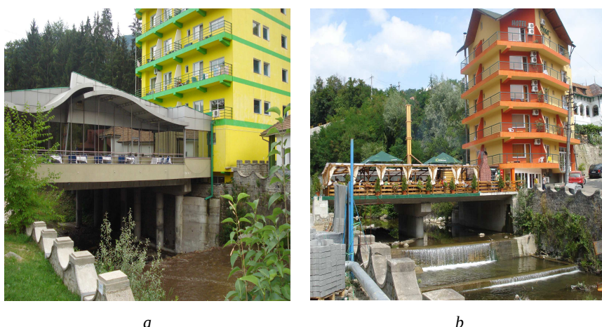
Fig. 5. The deterioration of the river bed Băile Olănești spa resort: a) Hotel Central; b) Hotel Stogu (Source: Roangheș Ana)
